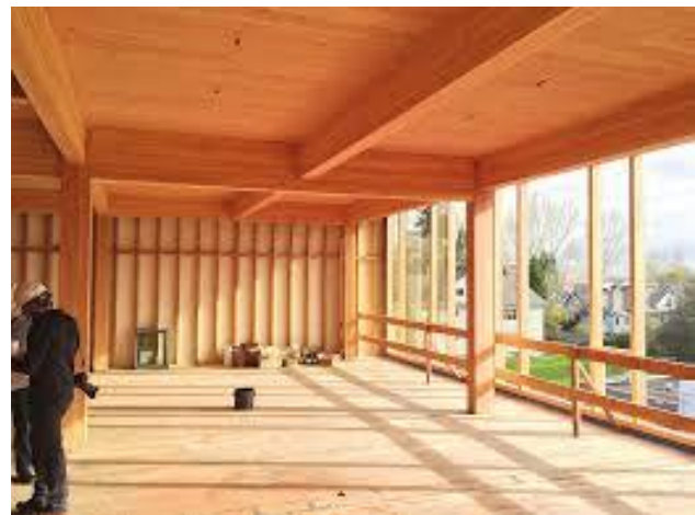
Figure 5. Mass timber building in Oregon under construction. Courtesy LEVER Architects.
